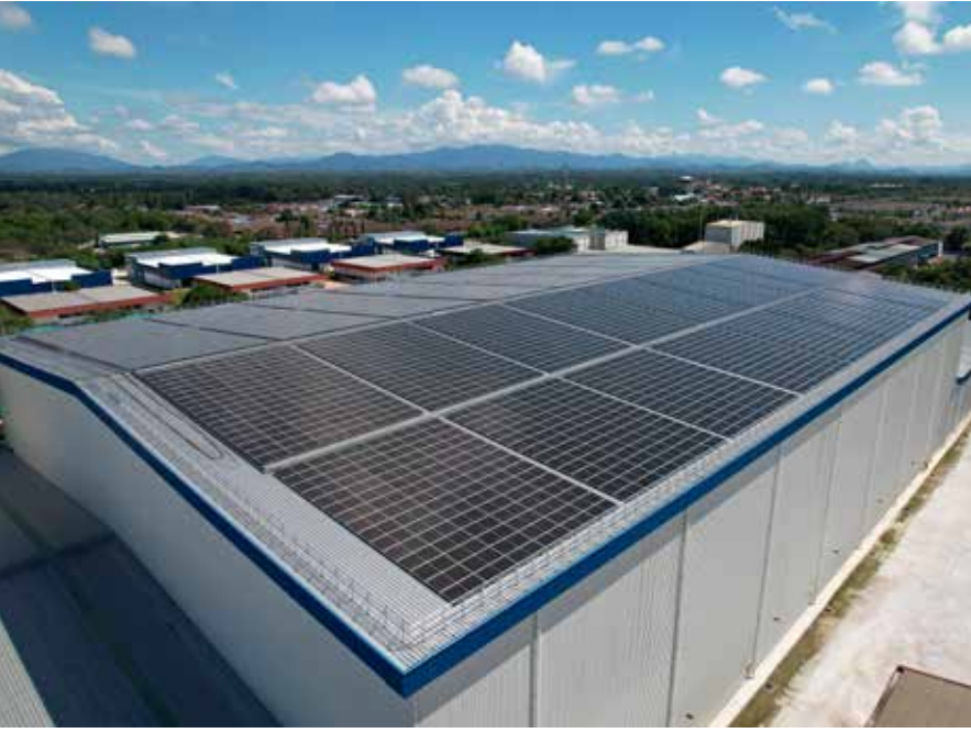
2 Solar panels on the building for the automatic storage and retrieval system
